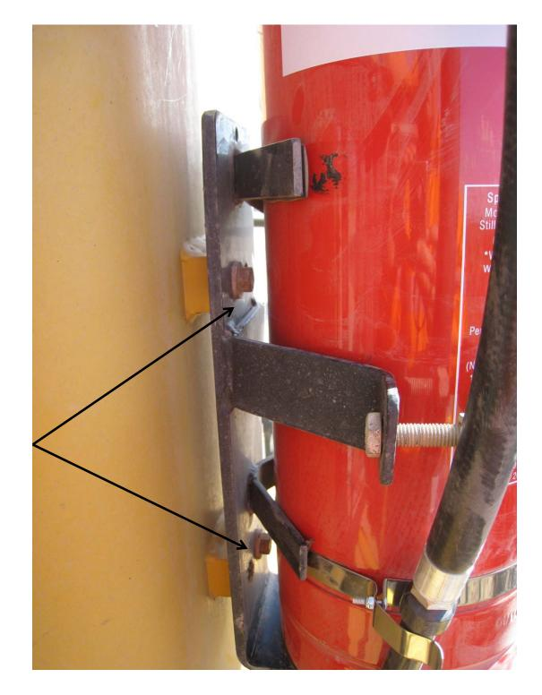
Burton – Checks found this FE with a corroded base – another potential bomb!
